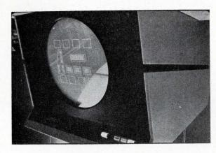
Interactive data terminal used in on-line CAD system. Several polycells can be seen in position.
