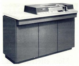
NCR's 420-2 optical journal tape reader, capable of reading 52 lines per second from the paper tape outputs of adding machines, cash registers, and accounting equipment.
