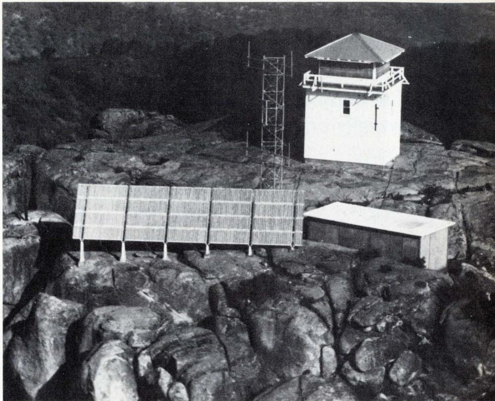
**5. The size of things to come?** Powering a communications link on a mountaintop in southern California is a solar-energy conversion array from Spectrolab. Approximately 900 square feet in area, the array produces well over 3 kilowatts of peak power. A big advantage of this kind of power source is that it can be left unattended.
