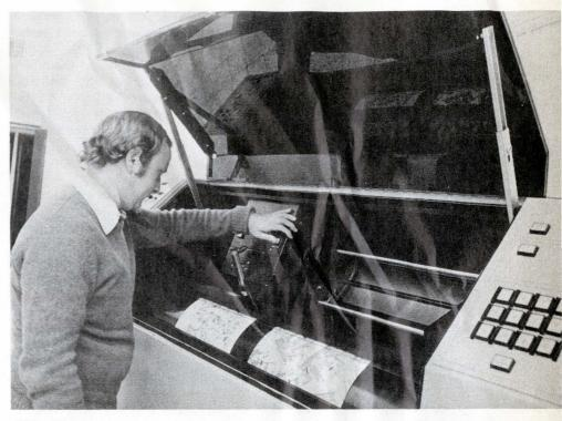
**Printer.** The optical scanner used in Sci-Tex Corp.'s design aid for the printing industry takes artist's pattern with as many as 12 different colors and converts it digital code. Design can then be manipulated via color crt.
