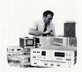
Troubleshooting a disc is a typical application for the new 1620A digital analyzer that scans parallel or serial bit patterns at rates up to 20 MHz
