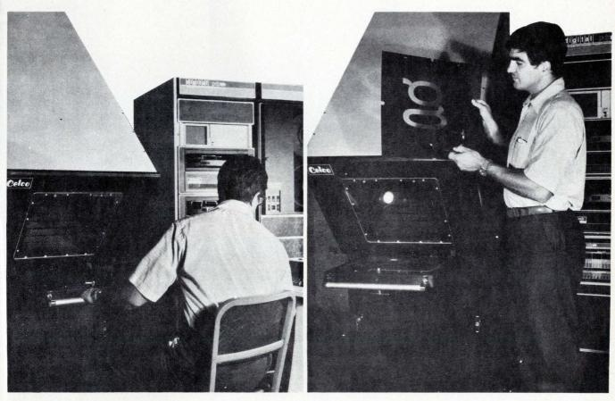
CELCO's Large-Format Scanner is a unique solution for automating the production of master fonts for a manufacturer of computer typesetting equipment. Scanning a 16-million point area, this system calibrates itself and reduces an artwork master 14 inches x 14 inches to a digital record in 16 seconds.
