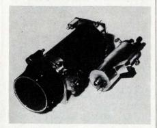
A UHF amplifier, for airborne equipment (right), was reduced in size and weight by using Dow Corning® 200 fluid. Only this unit produced full power over full frequency at an altitude of 100,000 ft.
