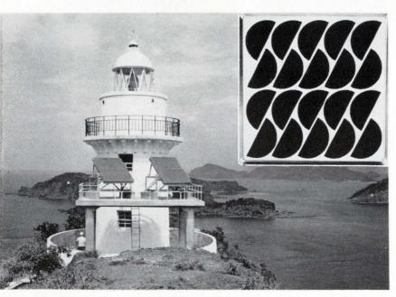
Alone under the sun. Unattended lighthouse off Japanese coast is powered by solar panels that generate 225 watts. Panels are built up of 20-cell packages shown in inset.
