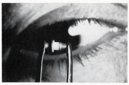
**Gallium-arsenide diode** is mounted in a metal-ceramic package; the pn junction oscillator can do the work of a low-power klystron tube 50 times as heavy.
