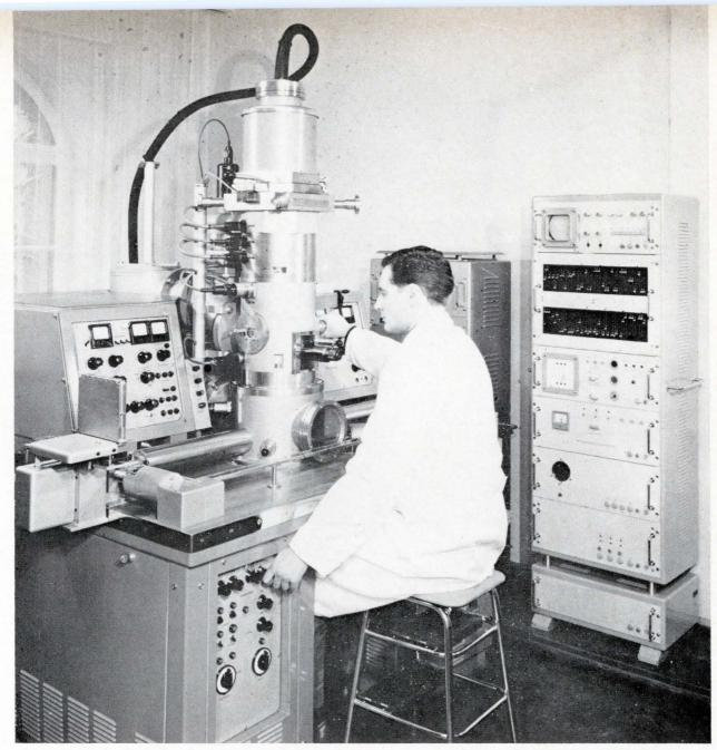
Electron-beam machining system trims thin-film resistors a a rate of one substrate every 2.4 seconds. Substrates are fed continuously into the vacuum system over the trac in front of the operator. The programer is at right.
