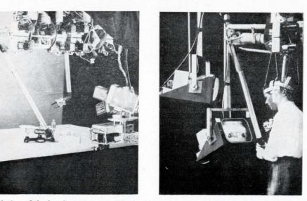
**Motion of the head,** as shown in this double exposure, produces a similar movement on a television camera and the monitor, providing a change of perspective for the operator of a remote-controlled manipulator. If the operator moves his head to the left, the camera that's trained on the "hands" of the manipulator (picture on the left) moves to the left and the tv monitor also moves to the left, remaining within the operator's field or view.
