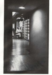
SIMULATED CAPSULE for remote control of Minuteman missiles. Low bridge tunnel, foreground, is protected—in the real nerve center—by an eight-ton blast-resistant steel and concrete door
