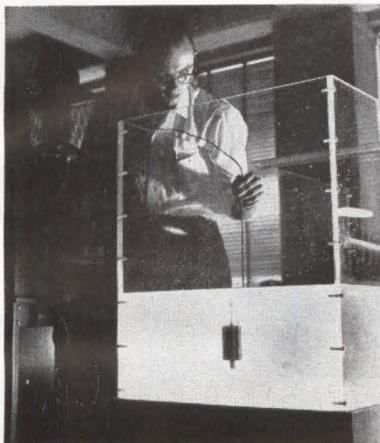
**PINPOINTING UNDERWATER** temperatures accurately is important in submarine sonar systems, since the speed of sound is affected by temperature. New transducer determines temperature to within 0.05 deg F
