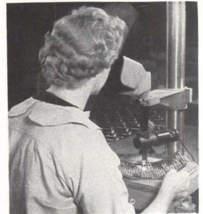
*OPERATOR locates target holes in terminal board in platter fabrication section of Raytheon missile plant. Holes will then guide drilling of additional holes*
