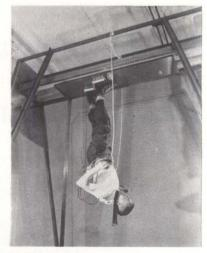
UPSIDE-DOWN MAN demonstrates possible space use for ceramic magnets that can have their poles reversed by switching circuit. Shoes can be used by astronauts during weightlessness in space. Magnets, developed by Westinghouse Electric, are being evaluated also for remote control, relay, memory and other applications
