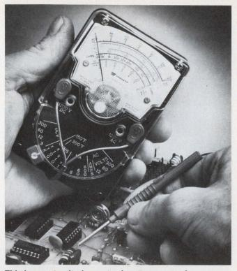
This low-cost volt-ohmmeter has two ranges for measuring temperature. The temperature probe in this Triplett instrument Model 100-T is a thermistor that measures from 50 to 300 F.
