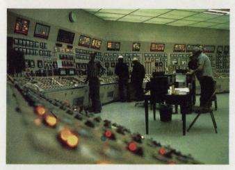
**Control room at Commonwealth Edison's Dresden reactor** in Morris, III., was built by General Electric. It displays data from sensors throughout the plant.
