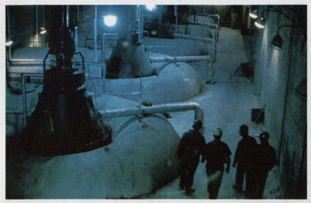
A computer displays diagnostic data from thermocouples on these giant pumps at the Commonwealth Edison plant in Zion. The pumps pull in 1.5million gallons of water a minute from Lake Michigan to condense steam.
