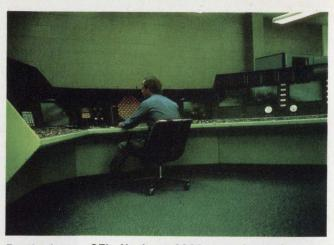
For the future, GE's Nuclenet 1000 control complex uses computer-driven CRTs to replace the hundreds of display meters that now line long control-room walls.
