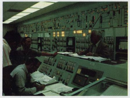
The delicate process of revitalizing used nuclear fuel is displayed in this control room in General Electric's Midwest Fuel Recovery Plant, Morris, III. A GE 4020 process computer logs the operation but does not control it.
