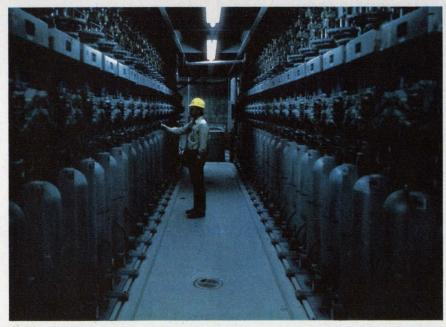
Hundreds of electronic sensors feed signals to these accumulator tanks of nitrogen. If conditions call for it, one or all of the tanks will release gas to insert the fuel rods into the core and shut down the reactor.
