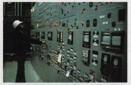
Waste disposal panel at the Commonwealth Edison plant in Zion collects data via Geiger-Mueller sensors from radioactive liquids throughout the plant. If preset limits are exceeded, the panel halts the operation.
