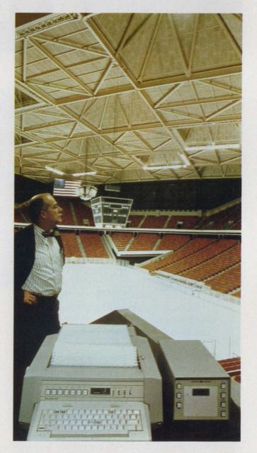
General Electric's Mark III computer network gets a workout in Atlanta's new Omni sports arena. James R. Fincher of Quo-Modo, Inc., operates a terminal that helps design the unusual Ortho-Quad truss structure.
