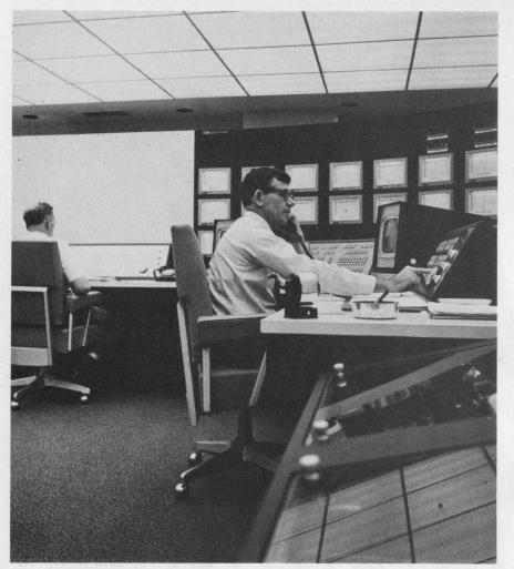
**Electric utility control system** built by Leeds & Northrup uses the company's Speedomax recorders on the wall to keep dispatchers posted on frequency and load conditions telemetered from key points.
