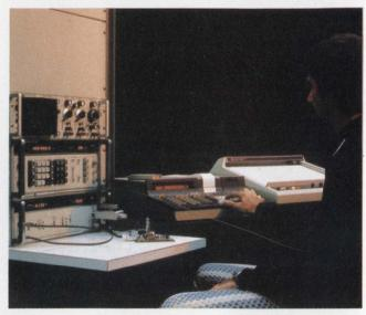
4. Automatic testing, data analysis and logging can be done by coupling a programmable calculator to programmable signal sources and measuring instruments. A programmable frequency sweeper and tracking detector, when added to a calculator, becomes a versatile network analyzer that is simple to program.
