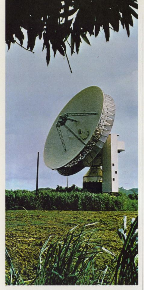
**Looming up out of a field of cane** at Cayey, Puerto Rico is this 85-foot earth station antenna. The station links the island with the U.S. mainland, Latin America, Europe and other Atlantic Basin points equipped with earth stations.
