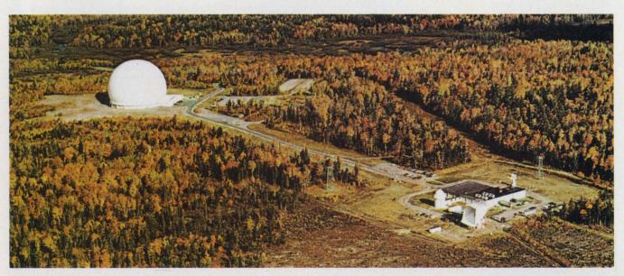
A huge 380-ton horn antenna is housed in this radome nestled in the autumn foliage near Andover, Maine. Originally built by Bell Telephone Laboratories for exper-
