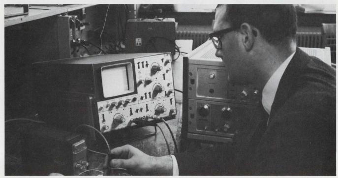
**Dual-trace oscilloscope** views dc-to-5-MHz signals with an accuracy of 200  $\mu$ V/cm. It
