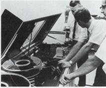
Plated disc memory with multiple read/write heads
