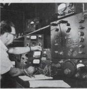
Screened room with precision test equipment assures close tolerance measurements for special coil characteristics. Intensive specialization in coil design and manufacture assures excellent operating results with a high degree of reliability.
