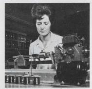
Special 16 Pi/30 KV windings for oil-filled, high voltage transformers : . . special coil samples are shipped within 1 to 2 weeks; production coil shipments start within 3 weeks after sample approval.
