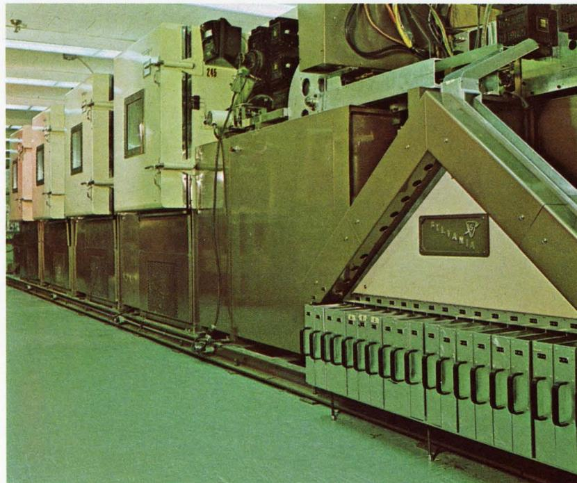
MR. ATOMIC tests each Sylvania IC in four temperature-controlled chambers.
