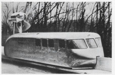
The French propellor-driven Aerotrain spins around its test track outside Paris. Clocked at 145 miles per hour, the French government and the French National Railroads are developing the Aerotrain for high-speed intercity passenger service (Session 58).
