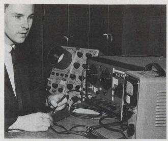
Measuring and testing the performance of IF amplifier that has simplified design. Page 38
