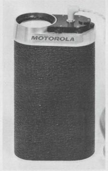
1. Motorola's experimental TV set is powered by four penlight cells.
