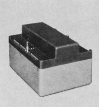
Customer: Control Data Corporation 128 x 64 x 12 capacity, temperature controlled stack for Polaris program
