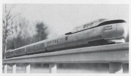
**Gas-turbine engines** will power this high-speed train designed by United Aircraft. Two such trains will be used in a demonstration project between Boston and Providence as part of the Commerce Dept.'s Northeast Corridor Demonstration program.
