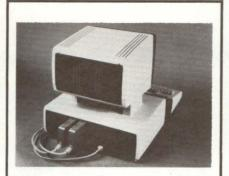
Fig 2 Four ports on System 45 hold a wide range of interface cards, allowing the user to expand the system and control or acquire data from as many as 20 instruments.
