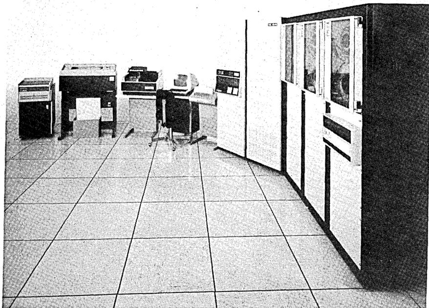
Systems Engineering Laboratories Model 32/55, shown above, is the firm's top machine until next month, when the 32/XX will be announced. One basic difference between the two models is the incorporation of user programmable writeable control store for the channels on the new machine.
