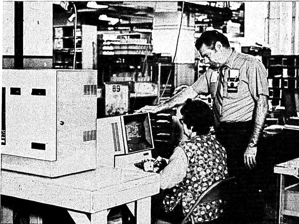
Variable length messages and inquiries are entered into the system at crt terminals such as this one in the stockroom. Such messages most often concern the flow of materials or orders rather than the status of a part being assembled.
