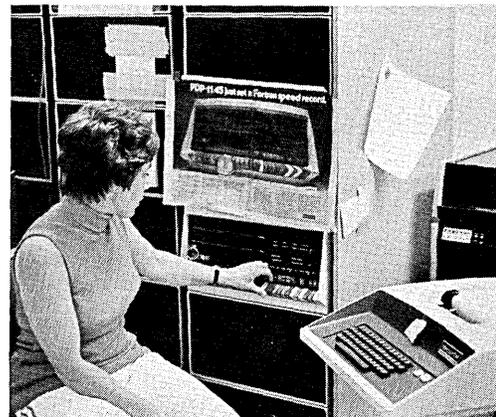
The minicomputer system which replaced the IBM 1130 was installed at a cost of approximately \$230,000. Time-sharing was implemented almost as an afterthought, but is now accounting for a greatly increasing portion of the machine time.
