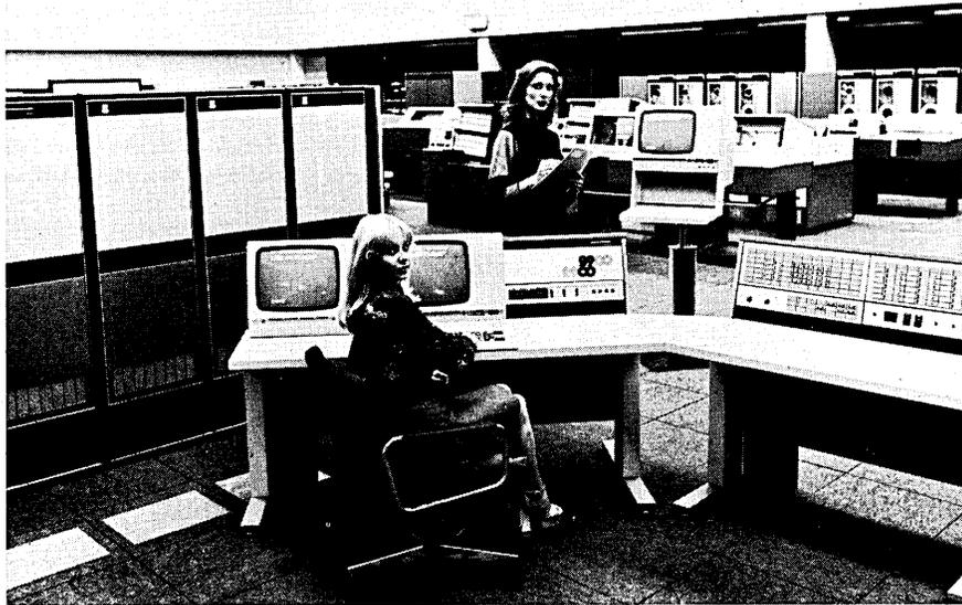
DELIVERY IN DECEMBER: ICL's 2970 system with operating console, order code processor at left and all the peripherals. Introduced last month, the first delivery is next month.
