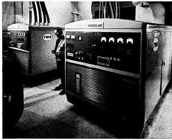
Two Solar gas turbine 800-kw emergency generators protect TWA computerized reservations center at Rockleigh, N.J.
