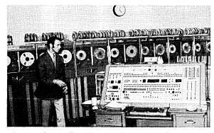
The Univac II, shown here at Computer Data Corp. in Gardena, has 2,000 12-character words of core and reportedly is still more reliable, though admittedly slower, than an IBM 360. This one has logged 558,571 hours.
