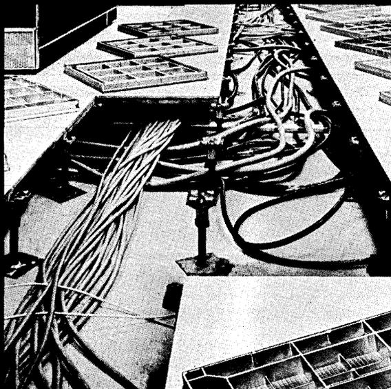
Elevated Floors provide full access to cables and ducts and a pressurized plenum for efficient, flexible, draft-free air distribution. Choose the best. A lightweight, aluminum panel, precision engineered, maintenance-free floor with all the reserve strength you'll ever need, from Floating Floors, Inc.
