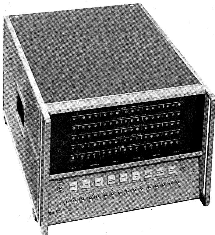
This new computer is the easiest to program and interface of all high-speed computers. It has 16-bit words, 4K expandable memory, 2 microsecond cycle time, plug-in I/O cards, multichannel priority interrupt, relocatable software and both FORTRAN and ALGOL compilers. Plug-in options including direct memory access and hardware multiply and divide are available. Peripherals such as high-speed disc memory and magnetic tape are standard. The price, with 4K memory and ASR-33 teletype: \$16,500.
