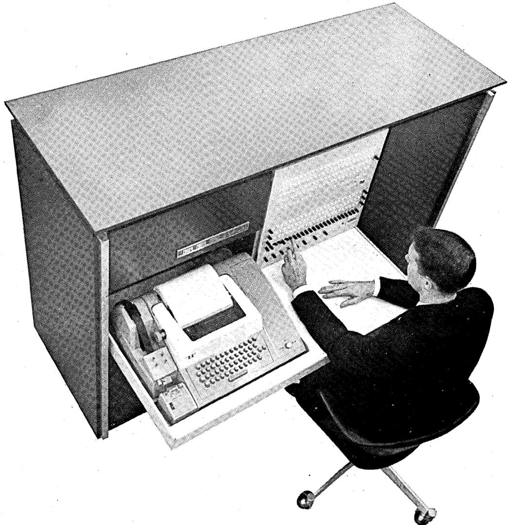
Our SEL-840A is the only computer in its class that offers an independent, concurrent, extended arithmetic unit (EAU) with a complete set of 22 additional hardware commands. The EAU performs 11 digit floating-point calculations as well as single and double-precision fixed-point calculations.
