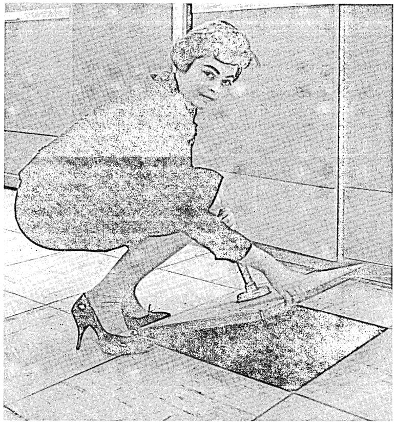
*Floating floors, which provide infinite access, are accessible and light.*
