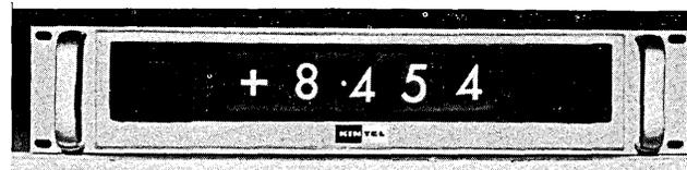
quirements are ¼ amp at 6.3 volts AC for each symbol or digit that is lit. Vertical space of 3½ in. is required in the standard 19 in. rack mount. Special models are available with up to nine individual readouts consisting of any combination of digits or symbols required. These digital readouts are designed for use with all types of digital converters and encoders. (Kin Tel, a division of CoHU Electronics, Inc., 5725 Kearny Villa Road, San Diego 12, California.)
