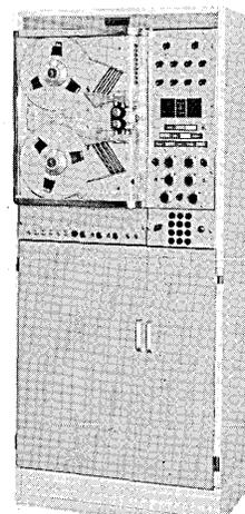
computing equipment. X-Y graphs of data recorded in digital form on magnetic tape is accomplished at high speeds. Used with any of the manufacturer's plotting boards, data can be presented in points, symbols, or continuous lines. Statistical charts of all types and many forms of mechanical drawings are drawn. For applications
