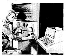
chine consists of one central processor and one input-output processor. Minimum memory capacity is 8,192 words, expandable to 131,072.
