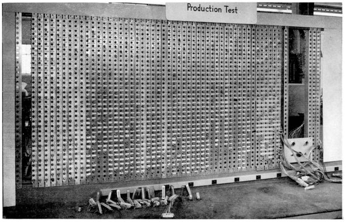
This piece of equipment checks the wiring of the digital differential analyzer made by Litton Industries, Beverly Hills, Calif. The 33 plugs at the bottom of the picture resting on the bench connect with the machine. The apparatus detects and locates open and shorted circuits which may occur in over 2000 soldered connections in the computer. (Figure 22)
