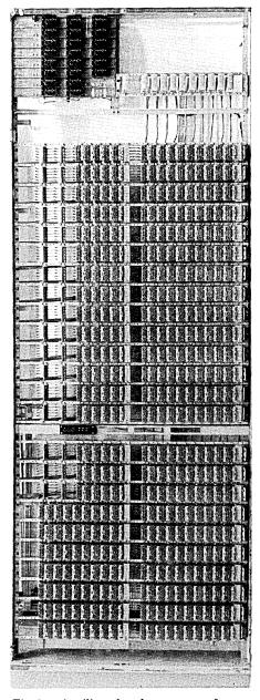
Fig. 31—Auxiliary decoder connector frame.
