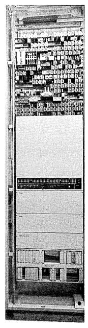
Fig. 37—Outgoing trunk testing system bay.
