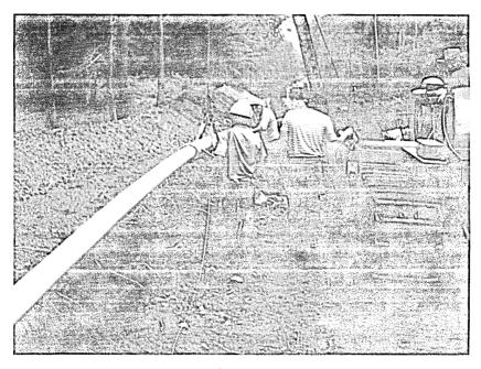
Fig. 8—Sheath being lowered into trench.
