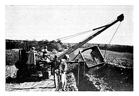
Fig. 8 - Backfilling and placing of shield wires.
