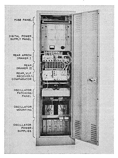
Fig. 15 — Rear view of reference frequency standard cabinet.
