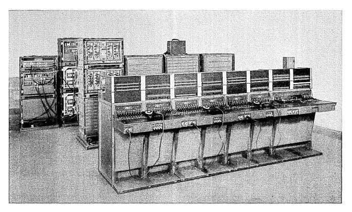
Fig. 3 — Typical three-position installation showing the preferred arrangement of switchboard and associated equipment.
