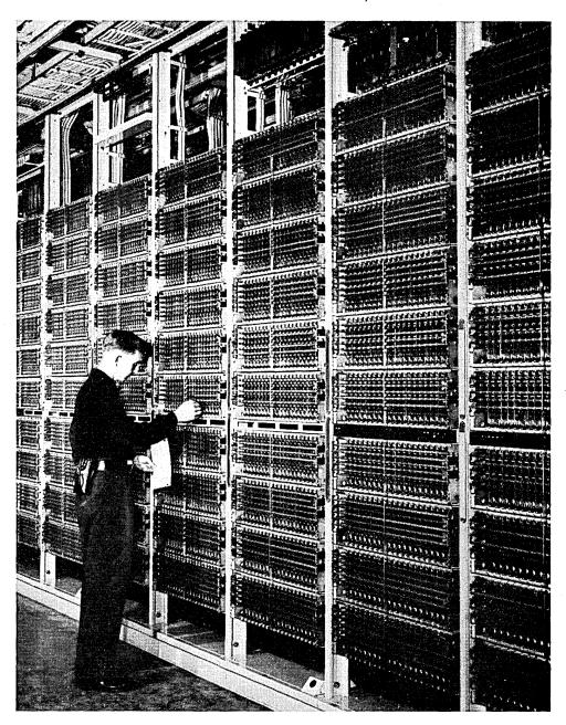
Fig. 18 — Part of a crossbar switching system.
