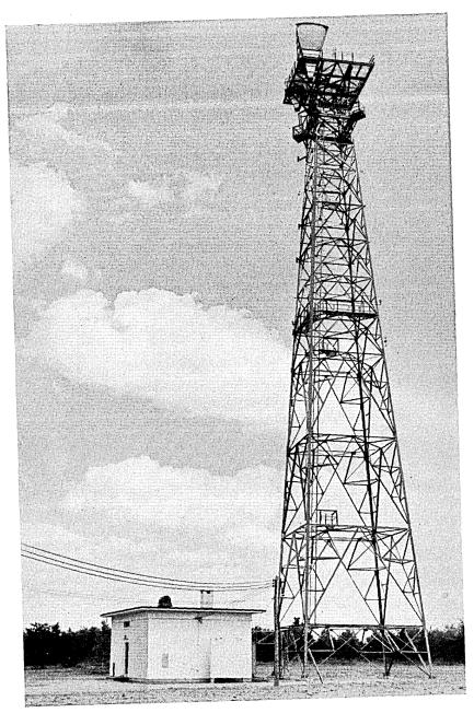
Fig. 13 — Microwave radio relay tower, Dawson, N.S.
