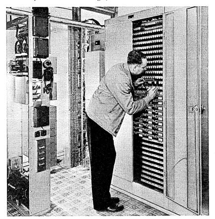
Fig. 19 — All-relay community dial office for telephone service in outlying areas. (By courtesy of North Electric Co.)
