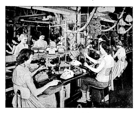
Fig. 7 — Assembly and testing of telephone sets.
