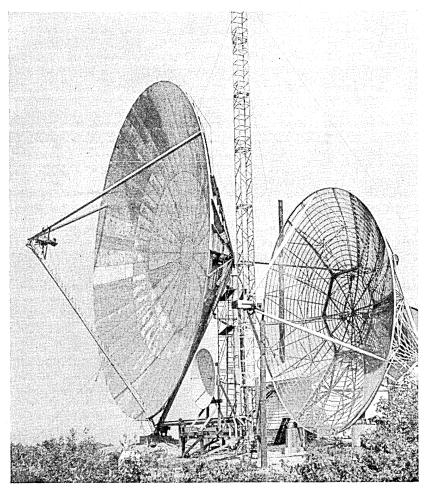
Fig. 9 — A view of the antennas at Crawford Hill used for beyond-the-horizon propagation studies and showing the 60-foot, a 28-foot and an 8-foot paraboliod, the latter between the two larger ones.
