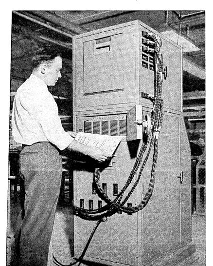
Fig. 5 - Rear view of Card-O-Matic test set showing insertion of perforated card.
